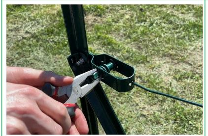
**Step 14:** Use pliers to twist the pin on the radisseur clockwise in order to tension the wire.
