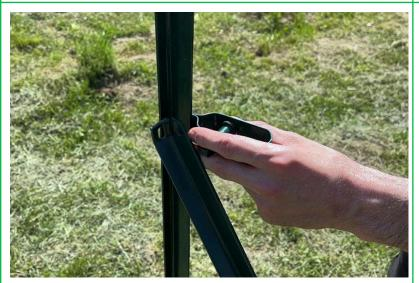
**Step 7:** Position the radisseur on the opposite side of the post, aligning it with the same hole as the strut.
