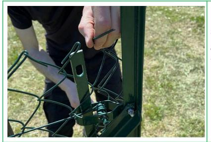
**Step 25:** Remove the excess mesh by gently untwisting one wire strand from where the cut is needed.
