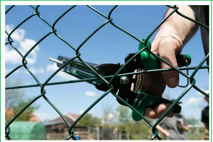
**Step 26:** Secure the tensioning wire to the chain link using hog rings.
