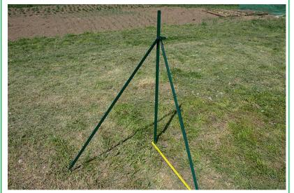
**OPTIONAL:** You can turn your end pole into a corner post by adding two struts at a 90-degree angle, providing extra stability at corners.
