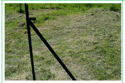
**Step 9:** The first end pole is now in place, supported by one reinforcement strut at the end point of the fence.
