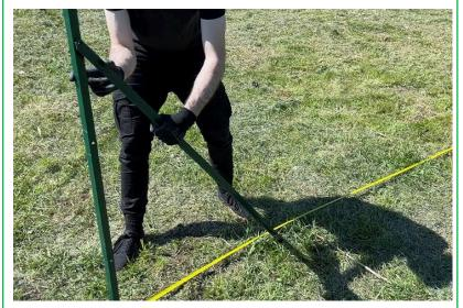
**Step 6:** Position the reinforcement strut, aligning its hole with the second hole down on the post.
