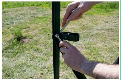
**Step 8:** Secure the strut and radisseur with bolts, nuts, and washers. Use two wrenches: one to hold the bolt and the other to tighten the nut.
