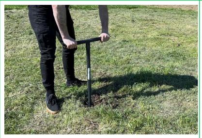
**Step 2:** Dig a hole for the first end pole using a hole digger.
