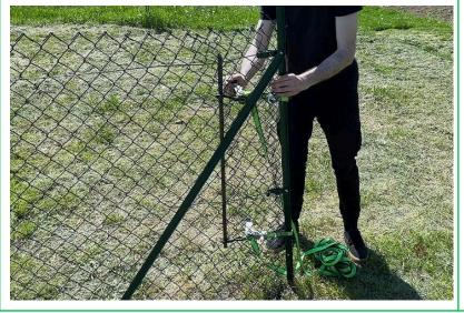
**Step 21:** At the other end, use a ratchet strap and an extra stretcher bar (or a rebar) to tighten the mesh. Gradually pull the mesh taut until it's properly tensioned.
