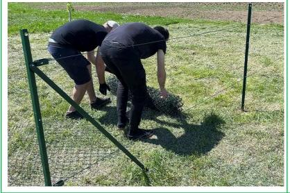
**Step 18:** Start unrolling the chain link along the ground. Be careful not to snag the wires as you go!
