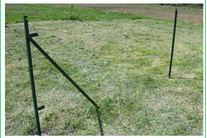
**Step 11:** Install the intermediate posts, which are not reinforced by struts, placing them at equal intervals between the end poles to keep the fence aligned.
