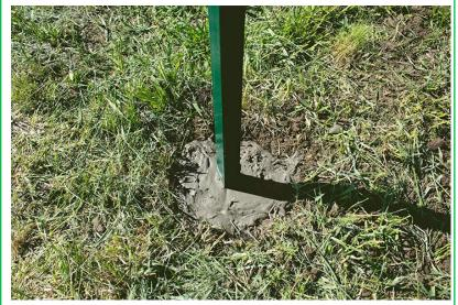
**Step 4:** Use concrete to secure the pole for added stability.
