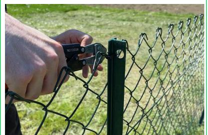
**Step 23:** Cut off the ends of the cable ties using wire cutters or scissors.
