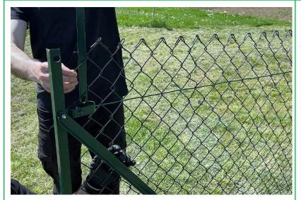
**Step 19:** Position the chain link fence near the end pole, then weave the stretcher bar through the mesh holes and the radisseurs.
