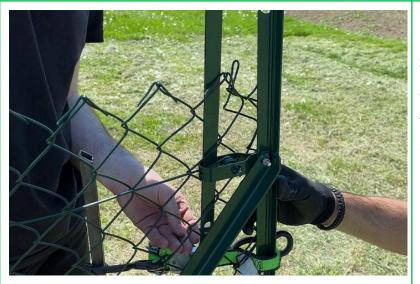
**Step 24:** Then, insert a stretcher bar as described in Steps 18–19 to secure the fence to the end pole.
