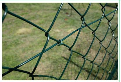
**Step 27:** Continue securing the tensioning wire along the entire length of the fence.
