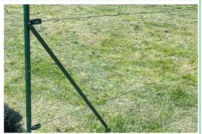
**Step 17:** Add a second line of tensioning wire along the bottom of the fence.
