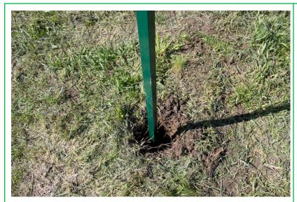
**Step 3:** Place the T post in the hole and make sure it's standing straight.
