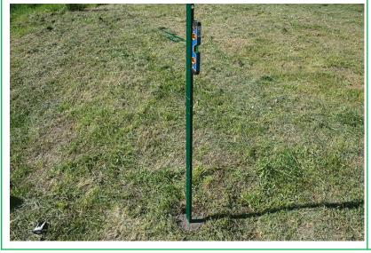
**Step 5:** Check with a spirit level to ensure the pole is straight before the concrete sets.
