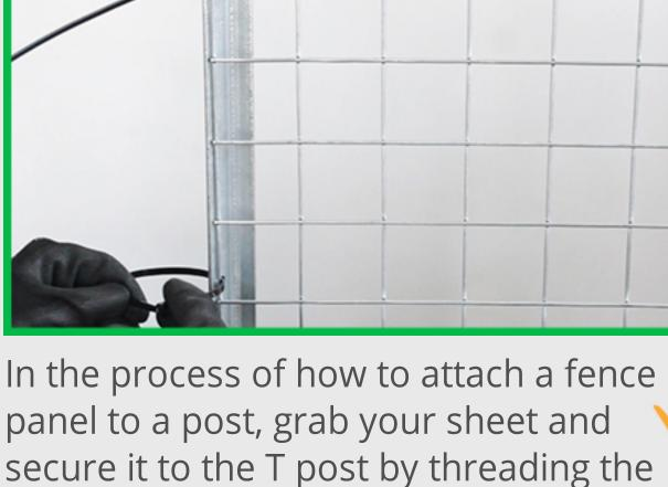
cable ties through the pre-drilled holes. **Cut off Excess**
