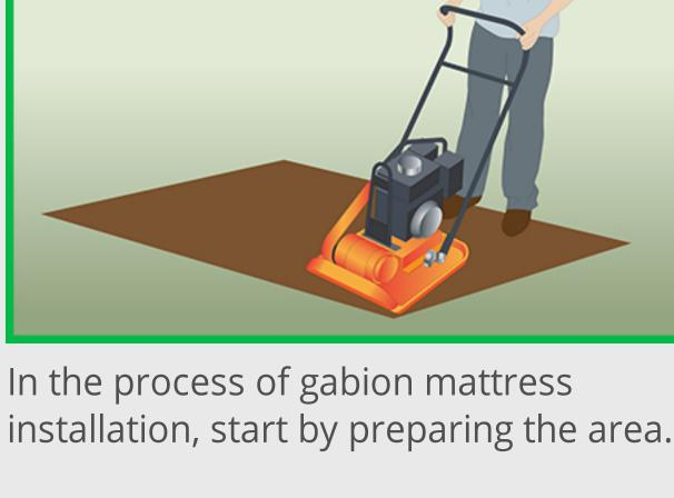
Remove any debris and make sure the surface is even and firmly compacted to create a solid foundation for the cage.
