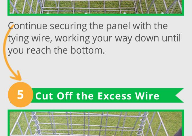
Use wire cutters to cut any excess tying wire once the panel is fully secured.
