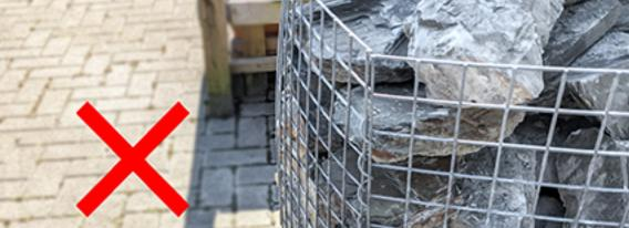
Bulging usually occurs when gabion baskets warp out of shape due to low gauge, increased force on the face or choosing the wrong shape of stones. This can be corrected by bracing the baskets with tying wire or by using corner ties.
