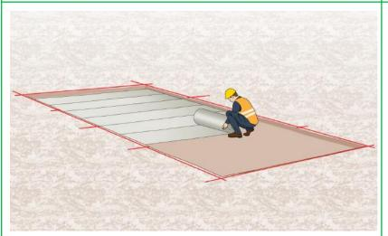
**Step 3:** Unroll <u>weed block geotextile</u> to stop weeds from growing up through the surface once the installation is complete.
