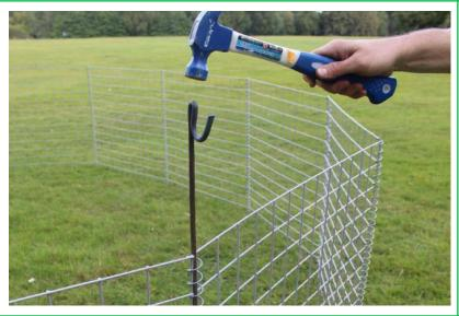
**Step 5:** Once it's in its final location, hammer the fence pin into the ground for added stability.
