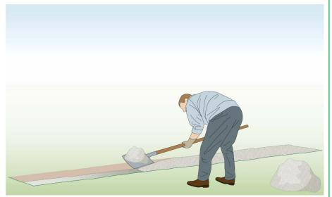
**Step 4:** Add a 20cm layer of gravel or basecourse on top of the geotextile.
