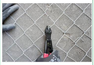
**METHOD A - Step 2:** Grab a mini bolt cutter and cut the marked strand from bottom to top.
