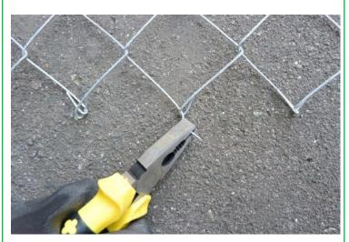
**METHOD B - Step 2:** Use a plier to unhook the top and bottom ends of the strand you just marked.
