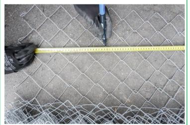
**METHOD A - Step 1:** Chain link has a woven construction so to make sure you follow the same strand when cutting, it's best to mark it from bottom to top.
