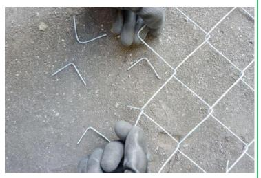
**METHOD A - Step 3:** Remove the small offcuts of wire that are weaved in the intact piece of chain link.
