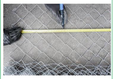
**METHOD B - Step 1:** To make sure you follow the same strand when unhooking the ends, mark along the length of the strand where you'd like your first section to end.
