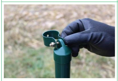
**Step 10:** Attach the strut clamp to the post cap using a bolt and a hex nut.
