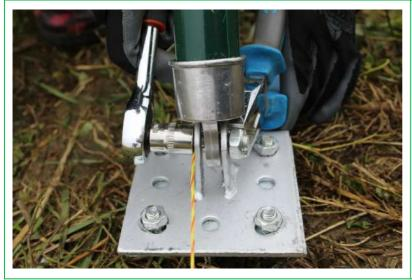
**Step 20:** Tighten the nuts on the angle post plate.
