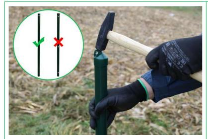
**Step 9:** Take one of the angle posts and add the post cap by gently hammering it on.
