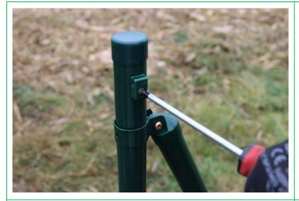
**Step 12:** Screw the fence clips on and add the post cap to the end post.
