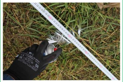
**Step 22:** Measure 2.5m distances from the first end post and mark the spots for your intermediate posts along the run.
