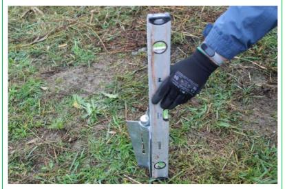
**Step 4:** Stop periodically and use a spirit level to make sure the post spike is plumb on all sides.
