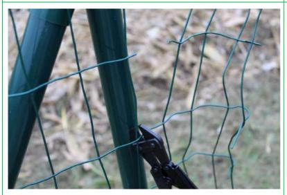
**Step 29:** Cut down any wires that are hanging off at the ends using wire cutters.
