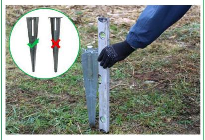
**Step 2:** Choose the location for your first post and stick a post spike into the ground. Insert the post driving tool into the post spike's hole.
