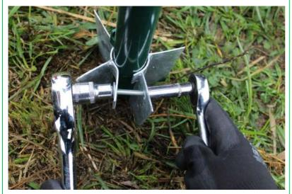
**Step 7:** Push a bolt through the holes of the post spike and add a washer and a hex nut to the outer end. Use ratchets to tighten it around the post.
