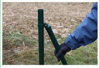
**Step 11:** Slot the clamp onto the upright end post.
