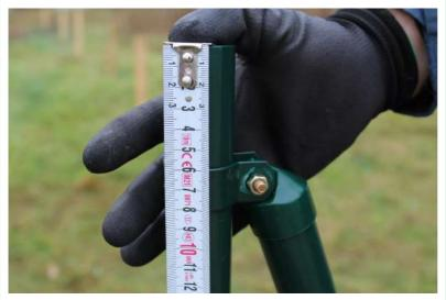
**Step 13:** Hold the clamp at a 6cm distance from the top of the end post.
