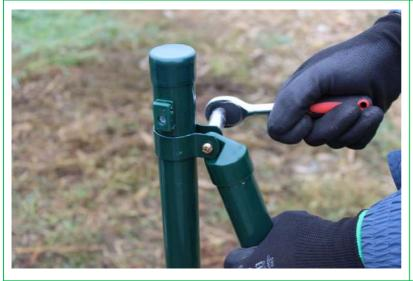
**Step 14:** Tighten the bolt with a ratchet until it's secure.
