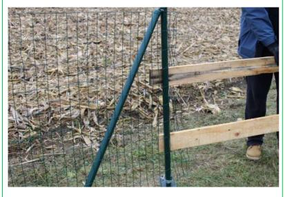
**Step 26:** To tension the fence, slot two wooden planks into the holes at the end and use the leverage they give you to fold the mesh gently back onto the post.
