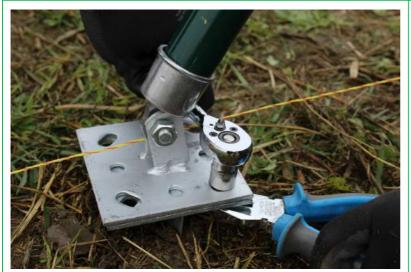
**Step 19:** Attach the angle post plate to the post spike plate with bolts and hex nuts.
