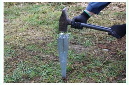
**Step 3:** Start hammering the post spike in deeper, hitting the post driving tool and not the spike itself.
