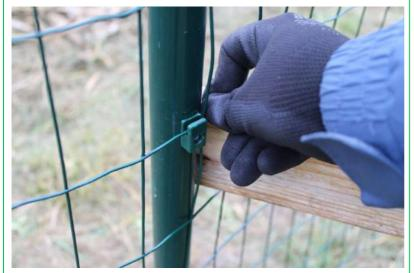
**Step 27:** When it's taut enough, lock the fence into place by slotting it into the mesh clips.
