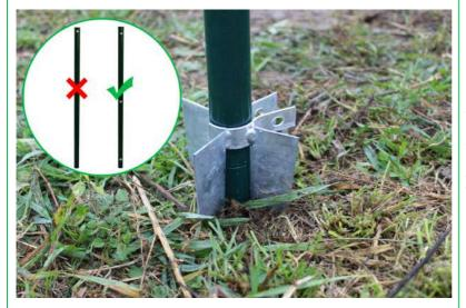
**Step 6:** Slot the first upright post into the post spike, making sure the holes for the fence clips face in the direction you'd like them to be.
