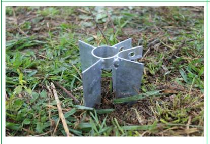
**Step 5:** Your post spike should be hammered in until the top of the empty slot in the middle is level with the ground.
