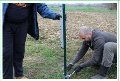
**Step 8:** Make sure the post stays completely plumb on all sides as you tighten the bolt.
