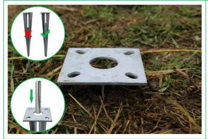
**Step 18:** In the position where the angle post reaches the ground, hammer in the post spike to the correct height (it should be level with the top of the first post spike).
