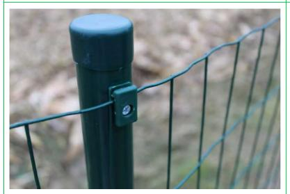
**Step 28:** Make sure the fence is clipped into every mesh clip (3x per post) at the holes that are in the same row under each other.
