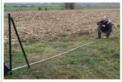
**Step 15:** Use a tape measure to measure and mark the end of your run (15m or 25m, depending on the length of your fence).
