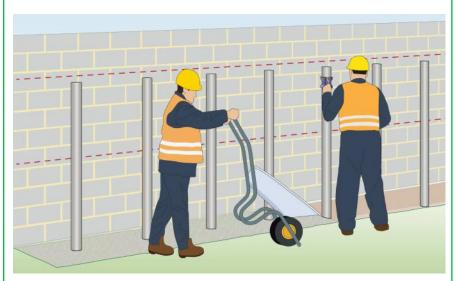
**Step 5:** Pour in your concrete to set the beams in place. Use a spirit level to ensure your posts stay vertical.
