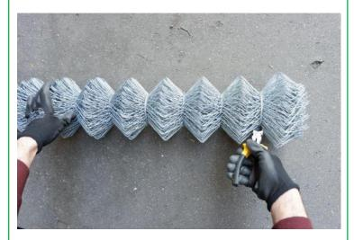
**Step 1:** Cut the tying wires that are used to fasten the roll and keep it from unraveling. Do this carefully so that you don't cut into the mesh itself.
