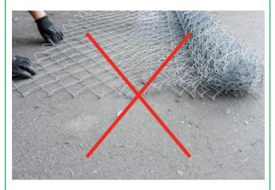
Make sure that the loose end of the chain link mesh is upwards and not down as it might get damaged if you unroll it that way.
