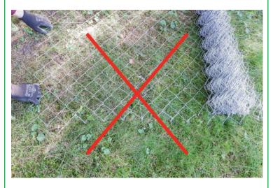
Avoid unrolling the chain link on soil or grass as it can get tangled up and undo the edges of the links.
