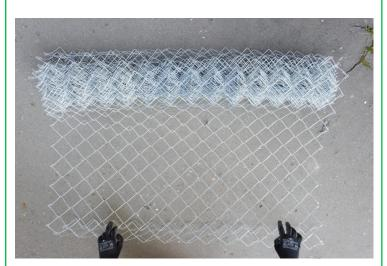
**Step 2:** Place the roll on the ground with the loose end upwards, facing in your direction.
