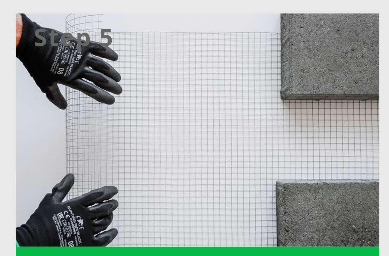
Grab the end of the cut down section and start rolling it out completely. Pull the mesh while doing this so that it straightens out because of the tension applied to it.
