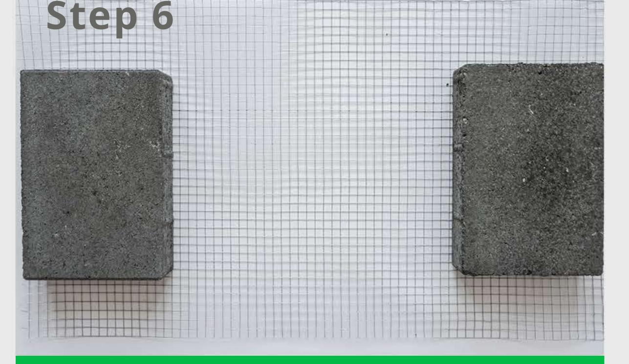
Roll out the mesh. Keep on placing heavy items where the wire mesh tends to curl back up. Leave them there until the mesh straightens out and keeps that shape.
