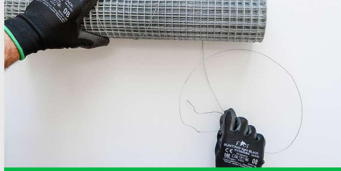
Place the roll on a hard flat surface. Start the process by unwrapping the mesh and removing the wire that holds the roll together. Have a partner help you by holding the mesh.
