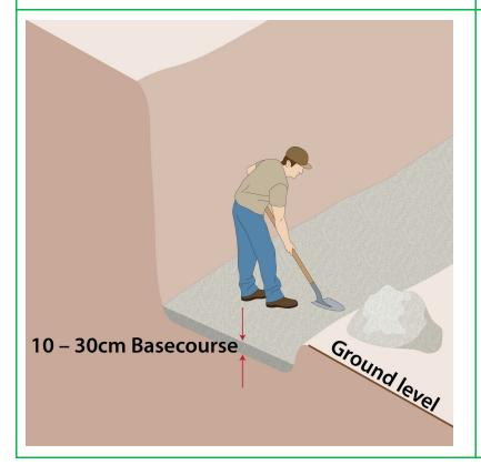
**Step 3 - Add Basecourse:** Add a layer of Type 1 basecourse made up of crushed Granite Limestone, Basalt or Gritstone.
