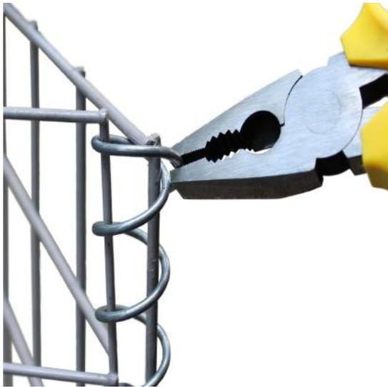
**Step 4:** To make the structure safer for your furry friend(s), fold down the top of the spiral connector so that no pointy wires are poking out of the top of the fence.
