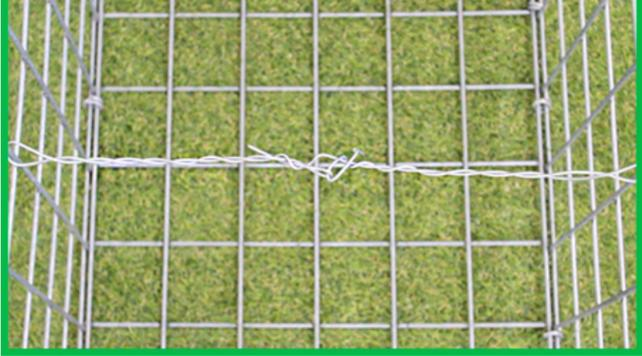
Start twisting the loop around itself with a screwdriver or a flat stone.
