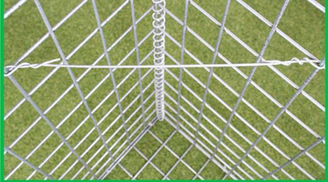
Use a piece of tying wire slightly longer than the gabion's length and connect the facing sides.
