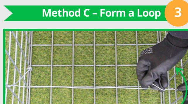
Twist the other hook as well. Make several twists to ensure the tie is firmly anchored.
