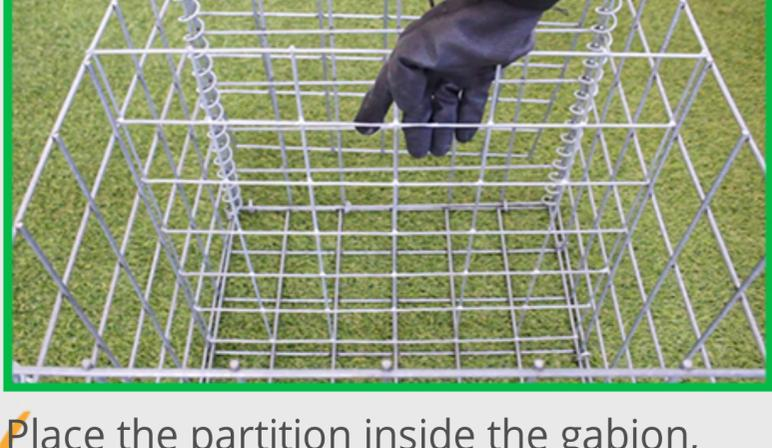
Place the partition inside the gabion, positioning it at the center of the basket's depth.
