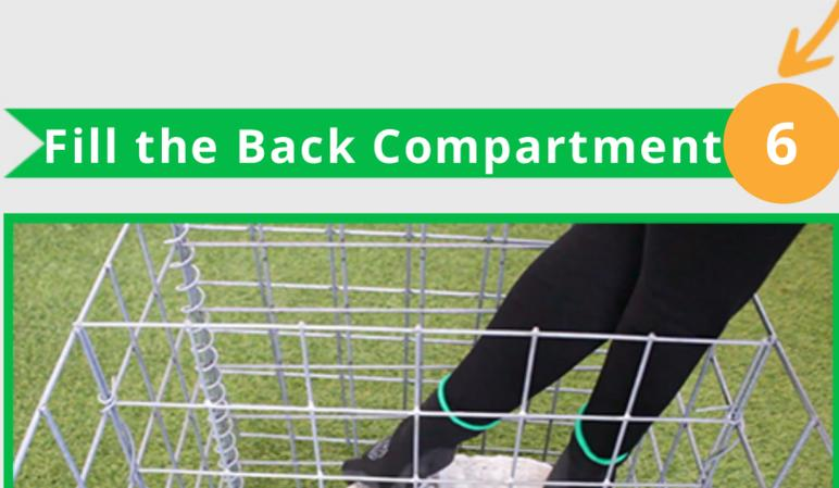
Start filling the back compartment with inexpensive rubble.
