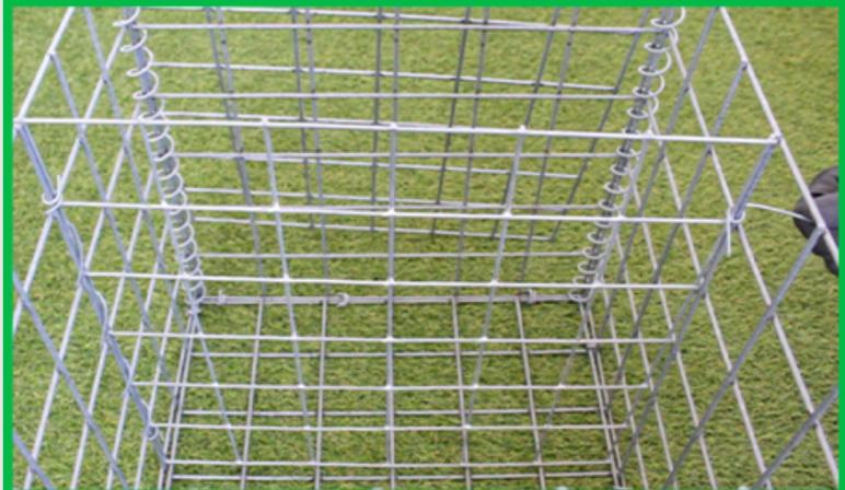
Start securing the partition to the top of the gabion mesh on both sides using the tying wire included with your basket.
