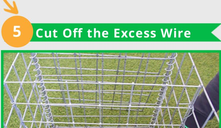
Use wire cutters to cut any excess tying wire once the panel is fully secured.
