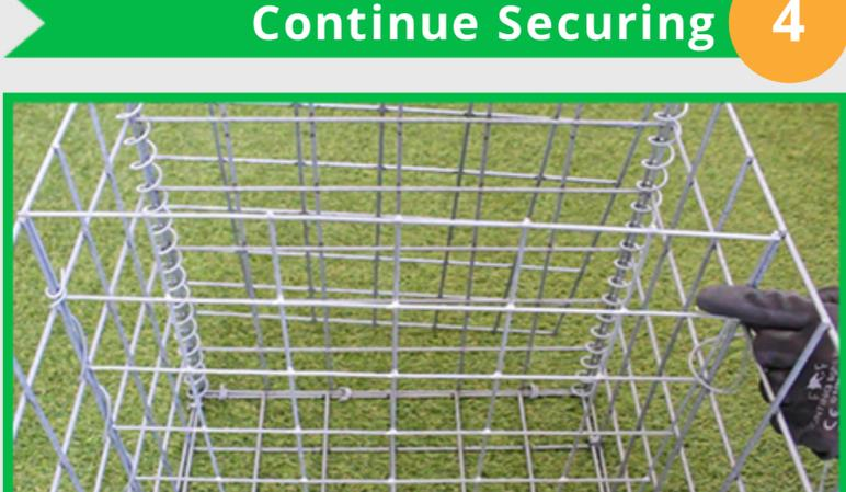
Continue securing the panel with the tying wire, working your way down until you reach the bottom.
