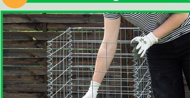
Use helicals to join the corners of the two baskets together. Make sure they enclose the corners of both basket's panels.
