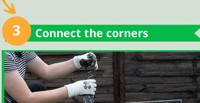
Measure the dimensions of the gabion panels and cut the helicals to match accordingly.
