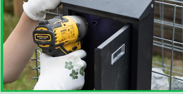
Place a wooden plank inside the gabion. Make sure the screw is right above a horizontal wire and the mailbox is positioned where you prefer.
