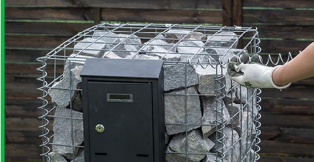
Secure your mailbox to the wood using an impact drill. Ensure that your mailbox is firmly fixed to the gabion and doesn't move.
