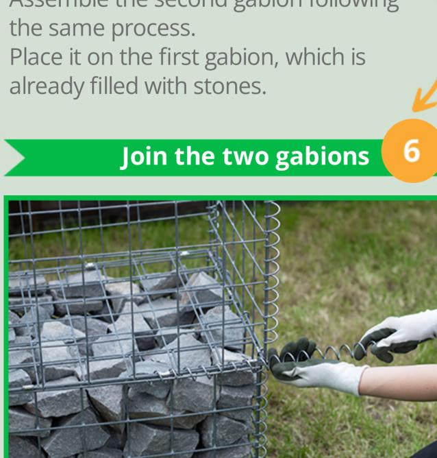
Assemble the second gabion following the same process. Place it on the first gabion, which is already filled with stones.
