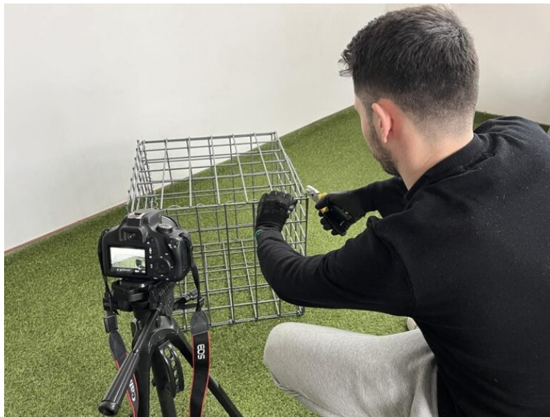
Erno lacing the gabion basket with lacing wire.
