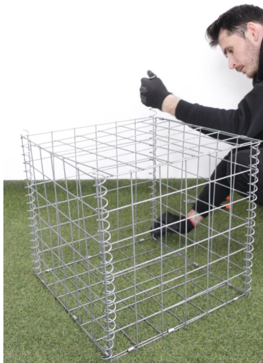
Erno securing the gabion with helicoil connectors.
